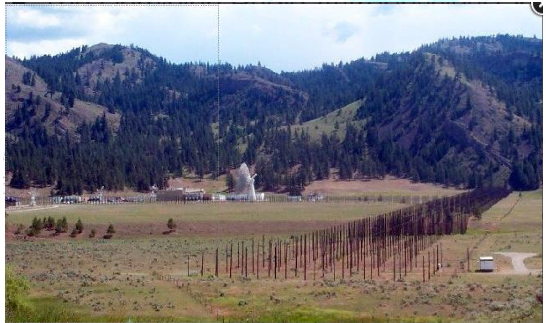
The 1,700 cedar posts of the 1.3-kilometre radio telescope. Source: National Research Council of Canada/Herzberg Institute of Astrophysics/Dominion Radio Astrophysical Observatory
